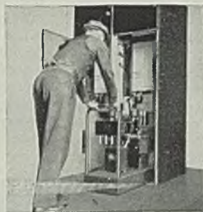
2. Removable Breakers — Easy maintenance
