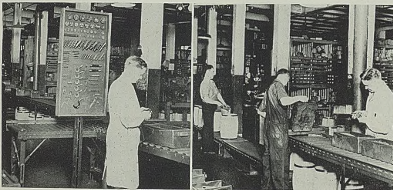
Fig. 3. (Left)—Gravity conveyor station in packing department where parts are inspected, before being packed. Fig. 4. (Right)—Note two levels of this gravity roller conveyor in the packing department. These permit work to be dumped from tote boxes at one level into shipping kegs on the lower level and so facilitate packing operations
