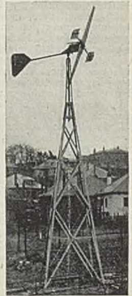
Typical wind-driven generating set in the Outer Hebrides
