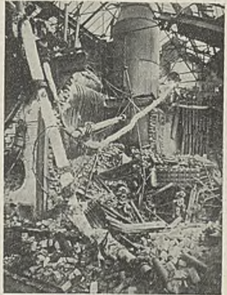
Bomb damage in boiler house at Eastbourne power station
