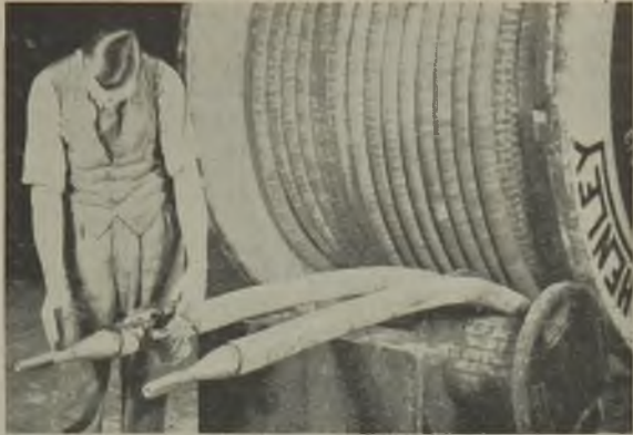
Preparing end terminations on a pair of finished cables
