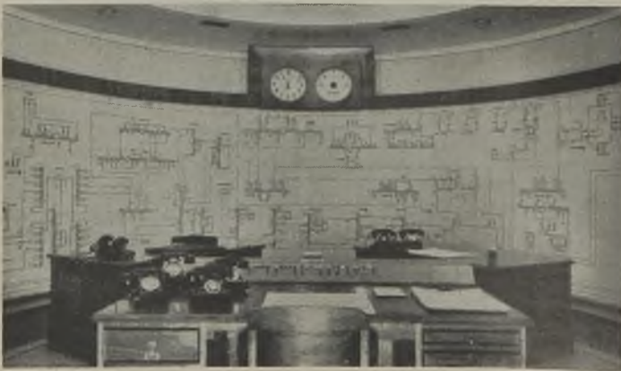
In the area switching control room is a cylindrically disposed main system diagram, transferred from Bankside, where it was arranged in one vertical plane
