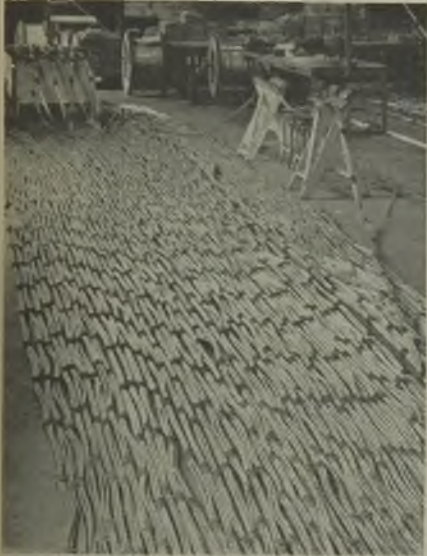
Electrode tails in course of assembly
