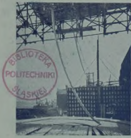
Coiling a length of many miles of H.A.I.S. Cable outside the HENLEY Cable Factory to await shipment.
