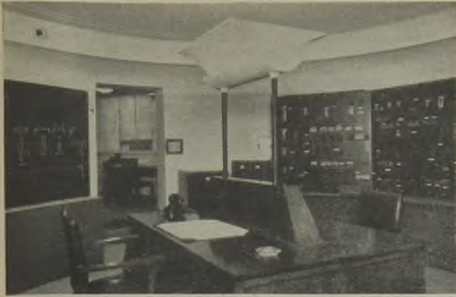
Calculator boards are used to check the duties imposed on the equipment with different switching arrangements, duties likely to be imposed on new switchgear, and for forecasting the distribution of load
