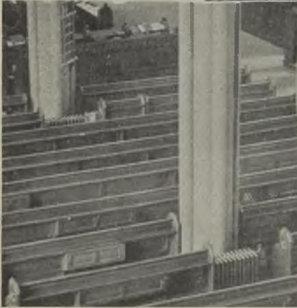
Above : Heating pipes, almost unnoticeable, have been run round the tops of the pillars to overcome the natural chimney effect. Left : Special low radiators at the base of the pillars for warming the centre of the building
