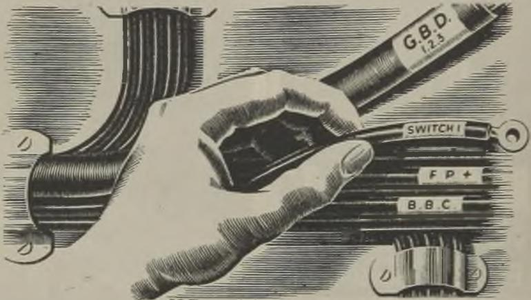
Ask the service man which "VISKRINGS" advantage he most appreciates and he'd have a job to choose. The swift identification by colour and wording. The knowledge that being impervious to oils and petroleum they will come out in just the same condition as they went in. The fact that having originally been fitted by shrinkage the diameter of the cable is not increased. These advantages and many more, have contributed to the enormous popularity of "VISKRINGS" Cable markers.
