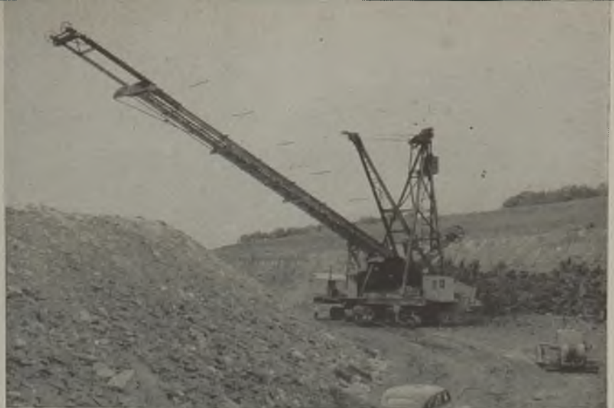
Spoil stacker at Georgetown enables a 5-cu. yd. shovel to act as an effective stripping unit.
