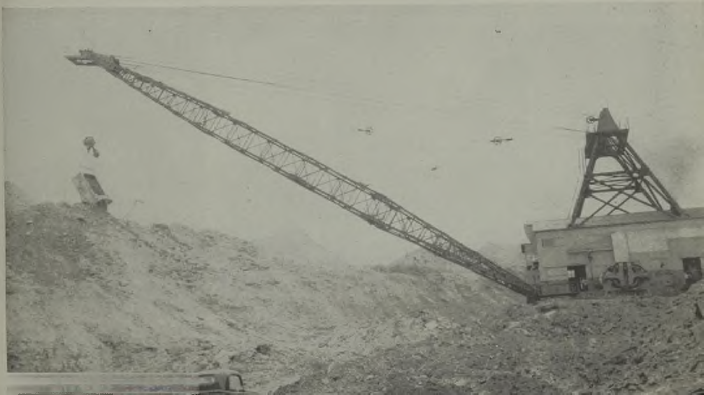
This 12-cu. yd. walking dragline handles up to 40 ft. of cover.
