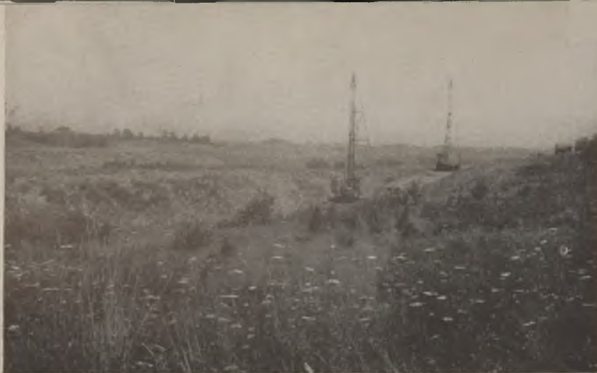
Two of the three churn drills working ahead of the 35-cu. yd. shovel where a new pit is being opened.
