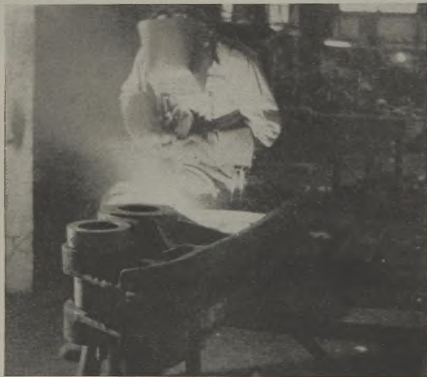
Fig. 4—New stiffeners are welded around the axle housing on loading-machine crawler frame which was originally cast in one piece. Old cracked stiffeners were burned out with a cutting torch
