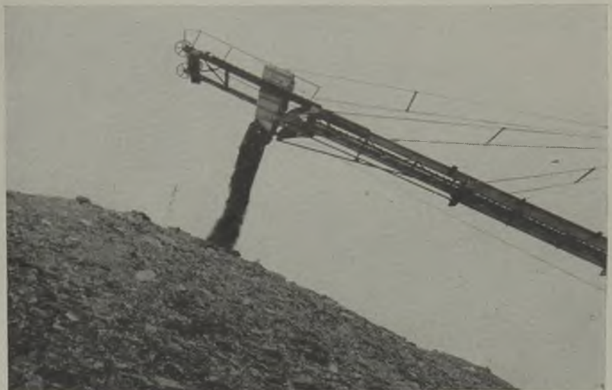
The 5-cu. yd. car of the spoil stacker makes two trips per minute.
