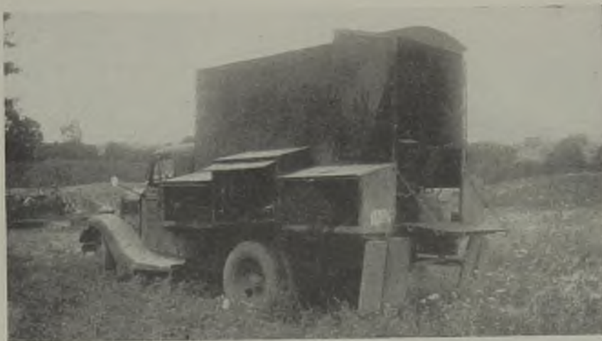
Equipment in the field lubricating truck includes a gas-powered air compressor and five outlets for various lubricants, each with a hose on a reel.
