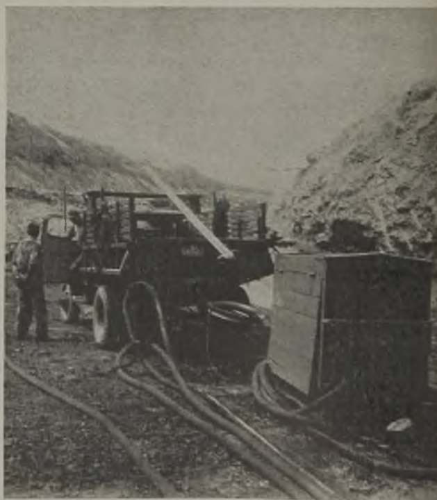
Truck moves the last junction box closer to the 35-yd. shovel.
