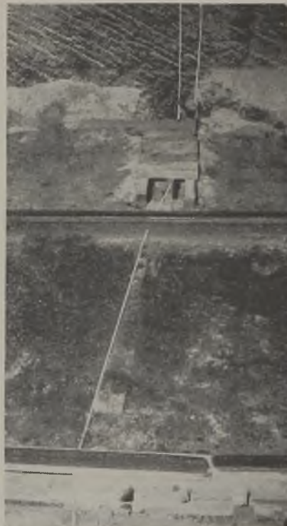
Broken wire or glass drops the weight, closing the switch to light the red lamps.
