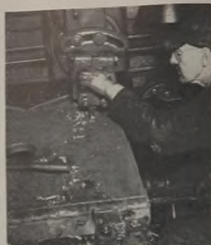
Once the plate is shimmed and clamped in place the operator takes it easy.
