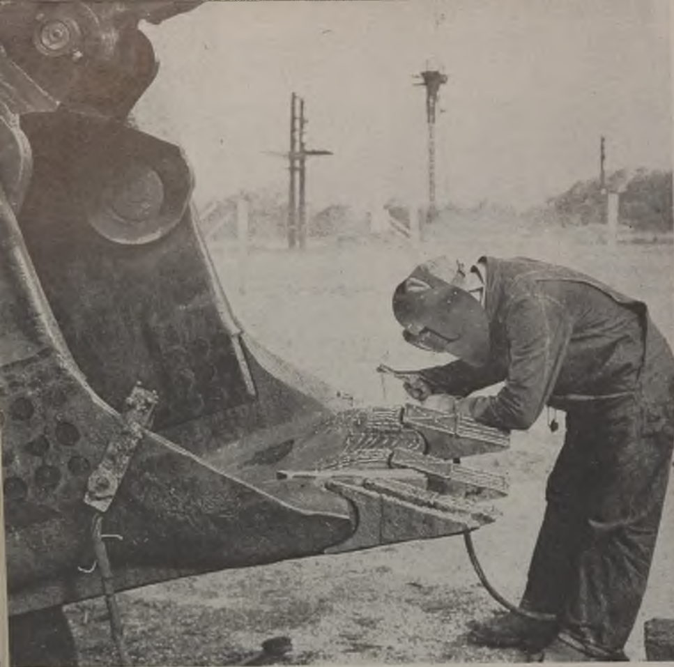
Fig. 9—All parts of the bucket subject to greatest wear are hard-faced before installation.
