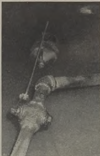
A gallon jug with cork stopper helps regulate the valve in accordance with the level of the water in the sump.
