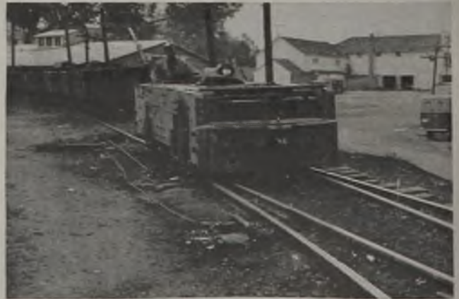
Here the locomotive has cut off from the trip and is coming through the switch. The trip in the foreground will throw the switch back to put the loads down the straight to the dump.
