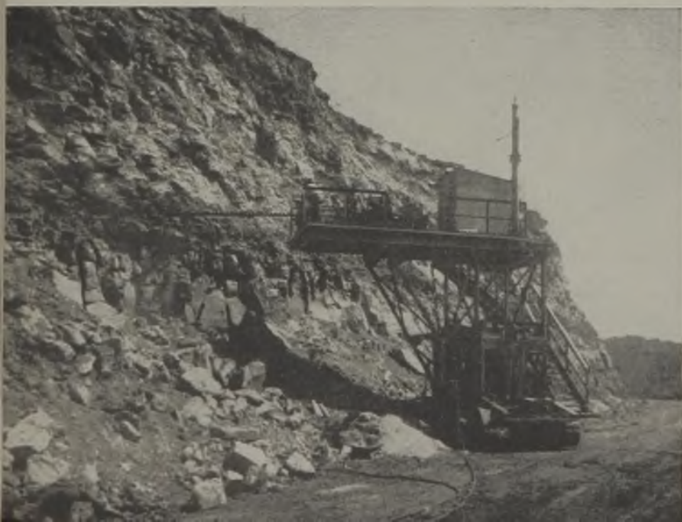
One of the two high-level drills assembled by Hanna to drill the sandstone strata lying high in the bank.
