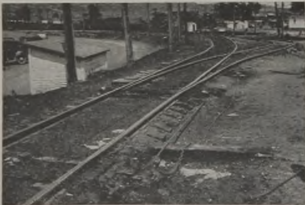
Ready for a trip to come in. The trip will throw the switch to permit the locomotive to take the right-hand track and then throw it back to allow the loads to go down the straight.
