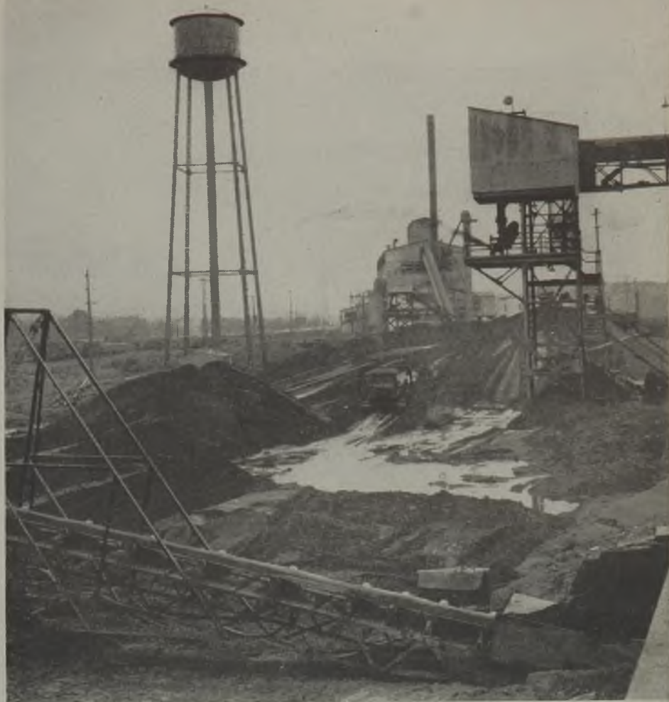
Loader-piler distributes the anthracite fines in the storage yard.
