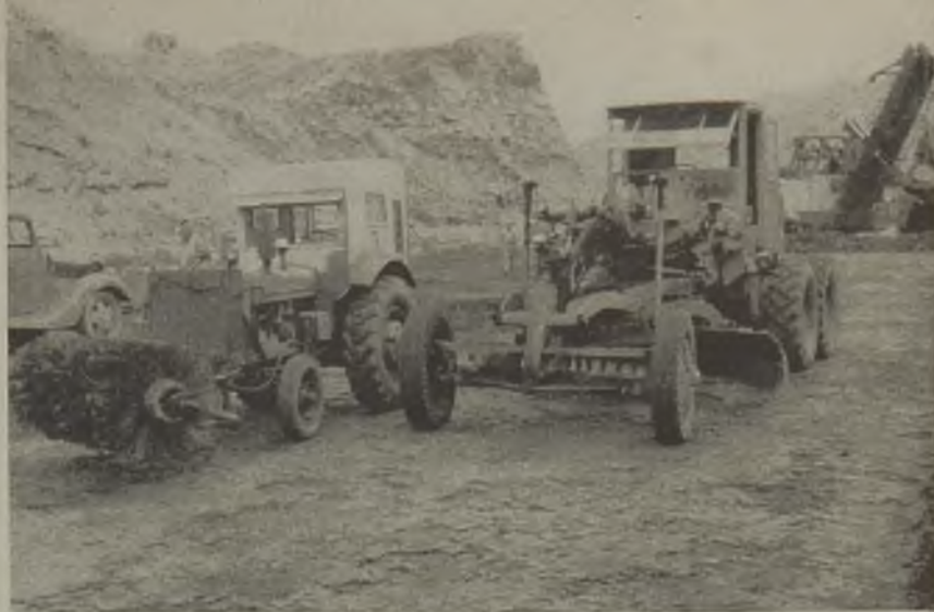
A scraper and sweeper work in tandem ahead of the loading shovel to rid the seam of all loose rock and dirt.
