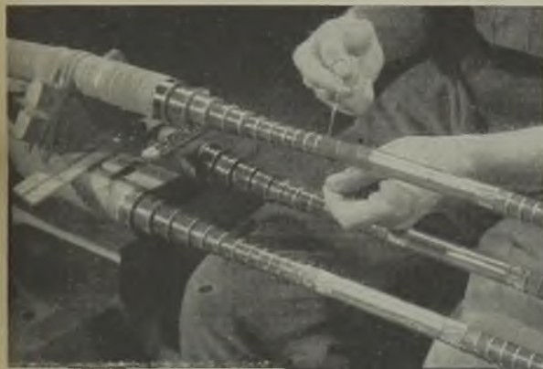
Joining 132-kV three-core 0.4 sq in. (120 MVA) impregnated pressure cable. Above is seen step formation of the cable dielectric after jointing with flush ferrules, with temporary spreaders maintaining core positions and temporary snuggers preventing disturbance of paper tapes. The right-hand illustration shows the three cores complete, tapered sections covered with lead-wire screen, internal pilot cable jointed and automatic pressure switch in position; gas communication pipes terminated on both sides near the top; lead sleeve partly pulled forward for placing in position and (on right-hand side) copper sleeve attached to travelling cradle
