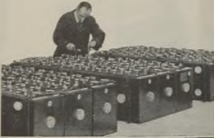
A Britannia Battery used for driving a locomotive belonging to an important ordnance depot.
