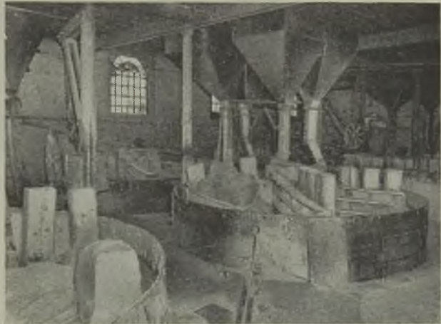
Pan room at Furlong Mills
