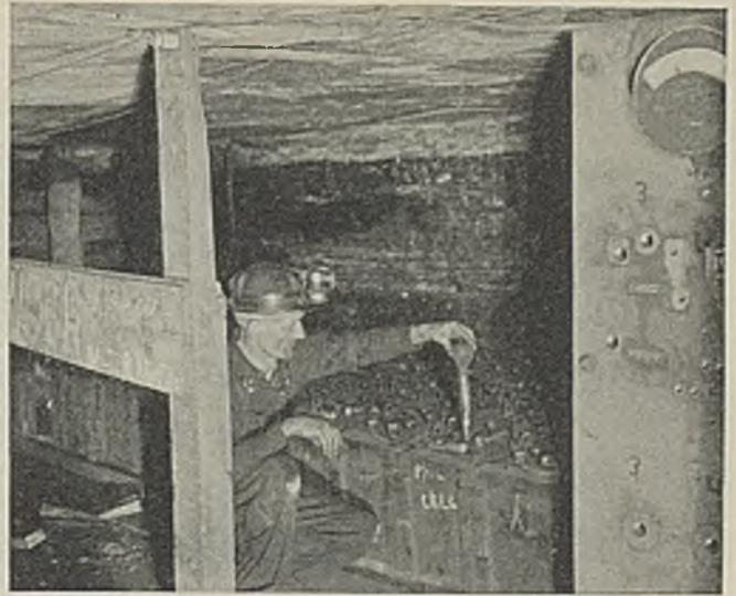
Left—A silent servant standing ready to cut 500 to 600 amp. from the peak load. Right—Mine Electrician Walker Renfro finds testing a few cells and adding water a simple task considering voltage benefit gained
