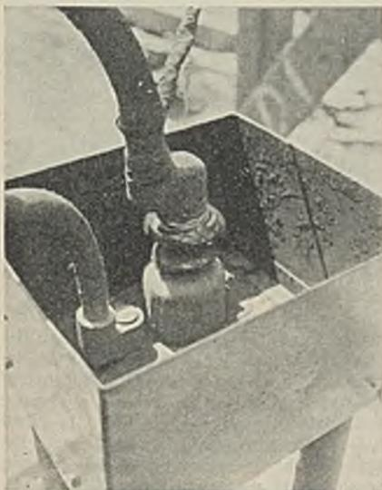
Suspension terminals rest on an Everdur plate. Metal sides were added as mechanical protection to the insulator
