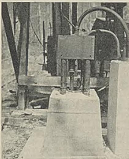
Between the car axle posts and below the guard can be seen the stuffing box and nut of the positive cable, also the seamless connector of the negative cable
