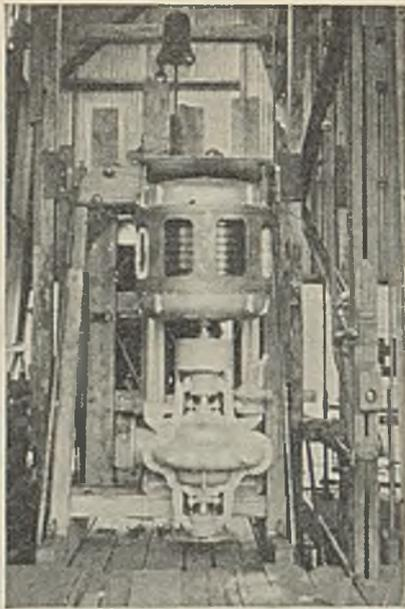
Mounted vertically, this pumping unit is about to go down the William A shaft
