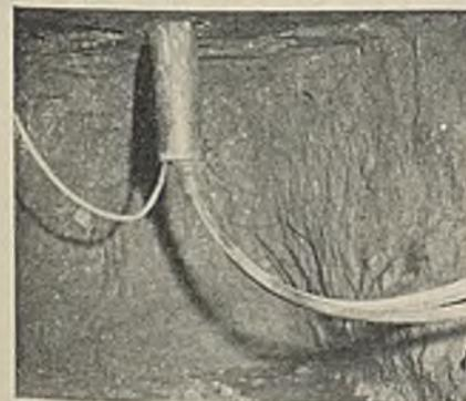
Casing and cables at the bottom of the borehole in No. 35 mine, No. 3 seam
