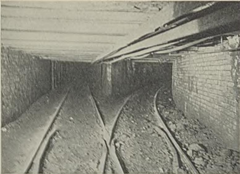
Steel beams and brick side walls and points are employed to protect main-line turnouts in the Clyde mines.
