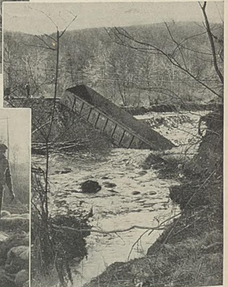
First of three railroad cars dumped in main channel through Lehigh Valley roadbed to mine breaches, March 22
