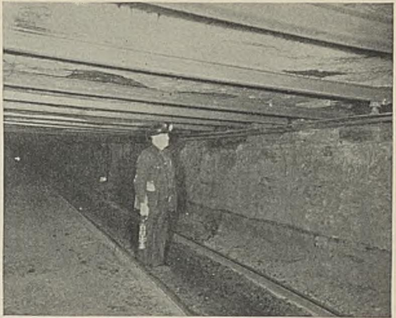
Henry Livingston, general mine foreman, No. 1 mine, inspects H-beams mounted in hitch-drill holes to protect a new stretch of 80-lb. loaded track. The 1,000,000-circ.mil feeder wire is suspended alongside the trolley wire on the right.
