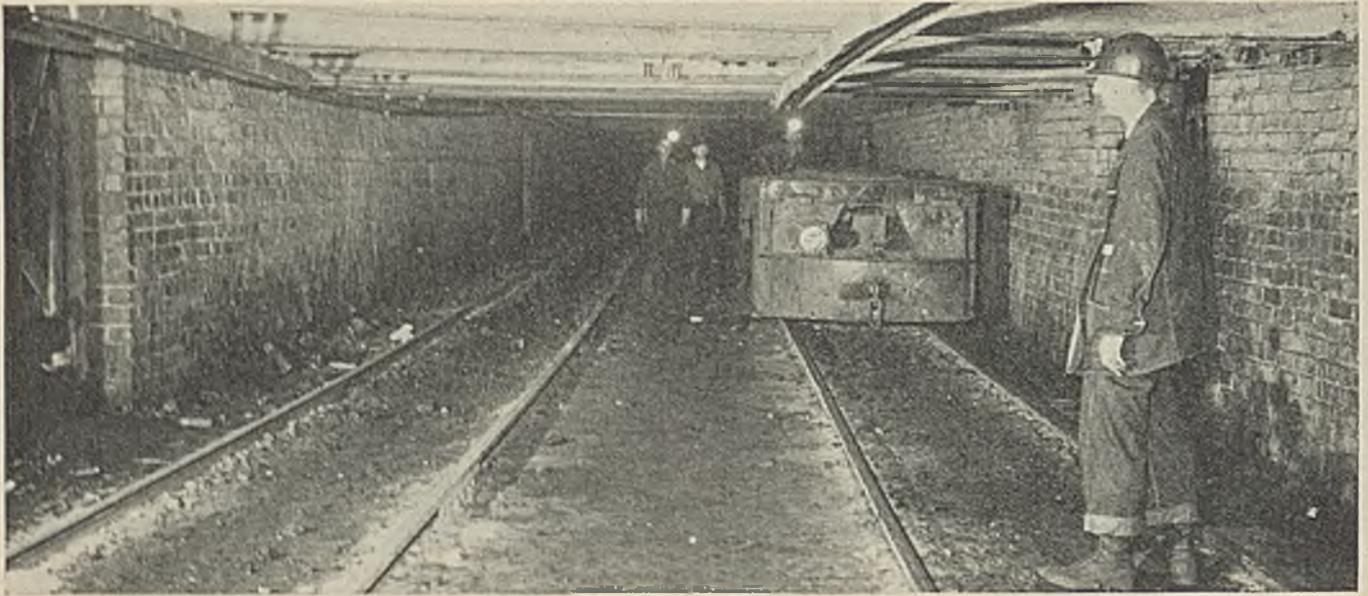
Inbye end of the double-tracked haulway at No. 1 mine. Roof support consists of steel I-beams on brick walls. At the left is the 80-lb. loaded track and at the right is the 60-lb. empty track with a haulage locomotive in the background and O. J. George, mining engineer, in the foreground. The creosoted ties have been in service since 1930 without a replacement.
