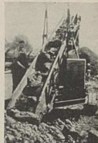
by the company. The unit is available in 25-, 30- and 35-ft. lengths with wheels or crawlers, gas or electric drive, gravity or vibrating screen, breaking bolt or B-G automatic load release and belt or chain-and-flight (drag-type) conveyors.
