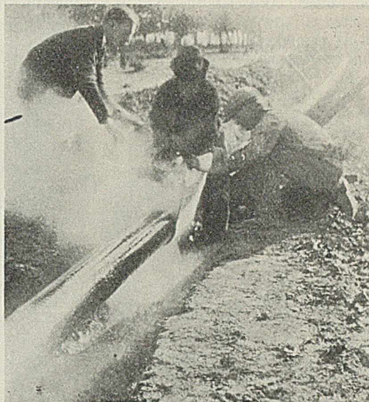
FIGURE 4. FIELD APPLICATION OF MOLTEN COAL-TAR PITCH COATING
