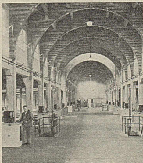
SOUTH FILTER GALLERY, OLD PLANT, MONTEBELLO FILTERS
