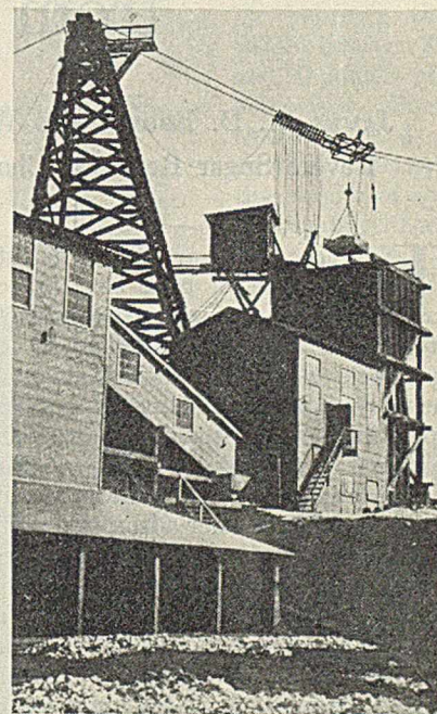
CABLEWAY DELIVERING FELDSPAR TO PLANT ACROSS THE RIVER, MINPRO, N. C.
