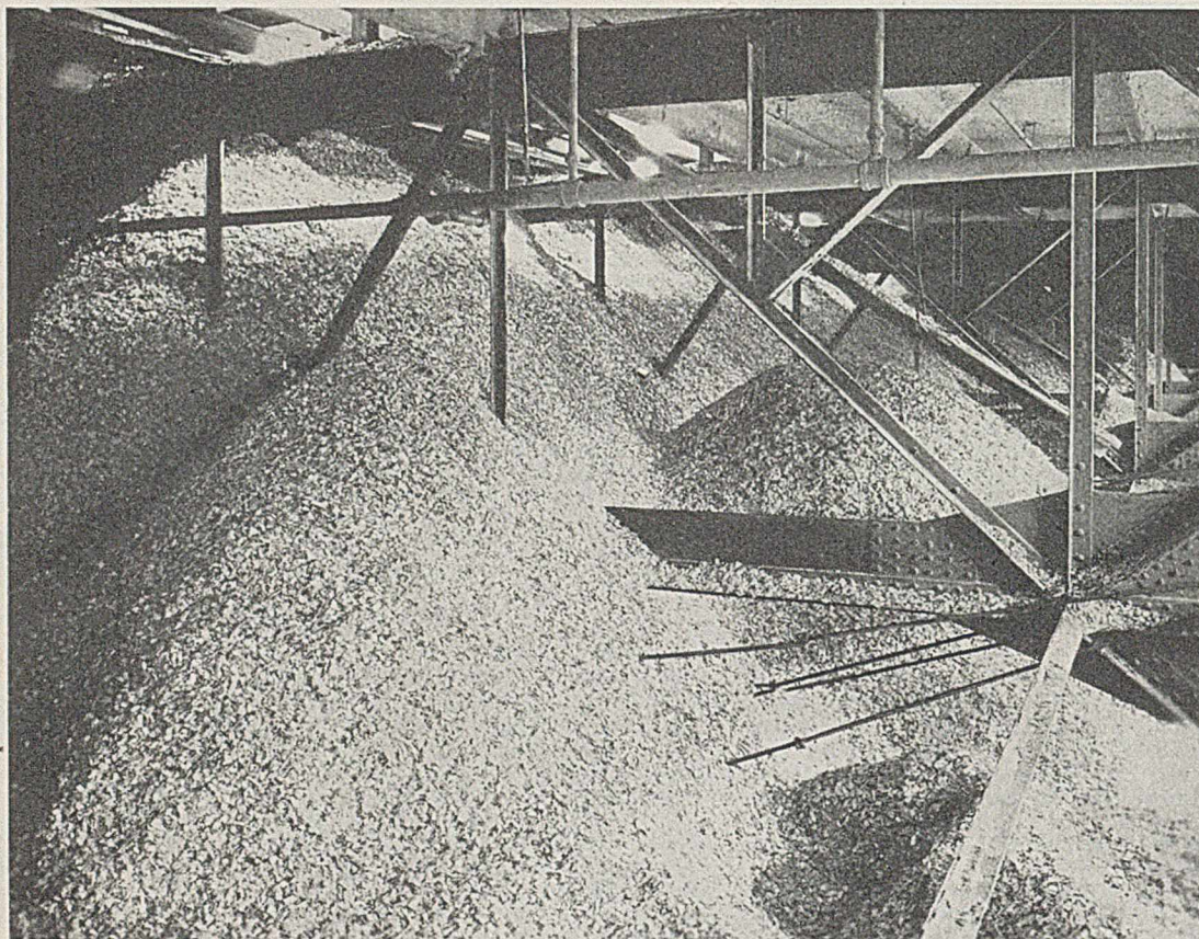
PORTION OF WOOD CHIP LOFT IN DIGESTER HOUSE
