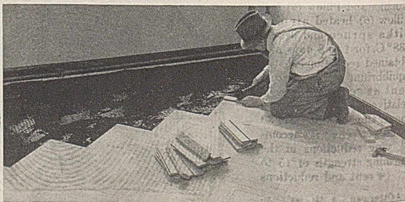
PARQUETRY FLOORING OFFERS POSSIBILITIES OF CHEMICAL TREATMENT TO MINIMIZE SWELLING AND SHRINKING
