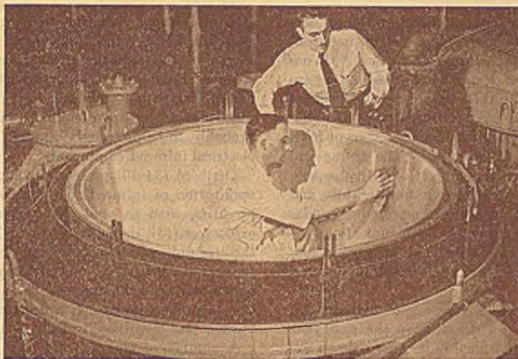
Rotor of the Five-Foot Molecular Still
