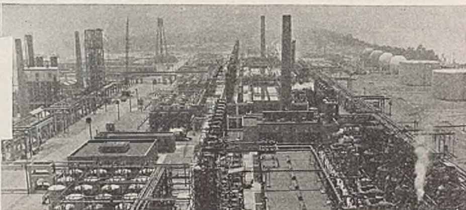
Butadiene and Power Plant, Kobuta, Pa.
