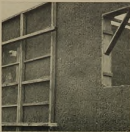
1 Eisenbeton in Lochblech-Schalung
