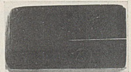
Figure 1. Stress-Corrosion Crack in 2-Inch Steel Wall of Autoclave
