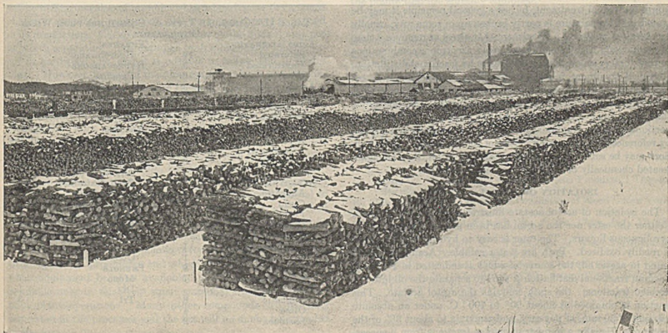
Plant and Portion of Reserve Wood Supply, Cliffs Dow Chemical Company
