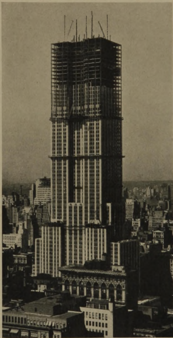
Empire-State-Building, New-York 85 Stockwerke, 85000 t Stahl, 6000 Stahlfenster Foto Ewing Galloway, N. Y.
