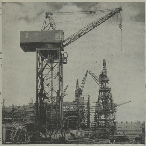
Above: An electrically operated I.B. Tower Crane (20 ton capacity at 60 foot radius) helps set production records at an eastern shipyard. Right: Note the patented Monitor-type cab which allows the operator 360° visibility on I.B. gas or Diesel locomotive cranes.
