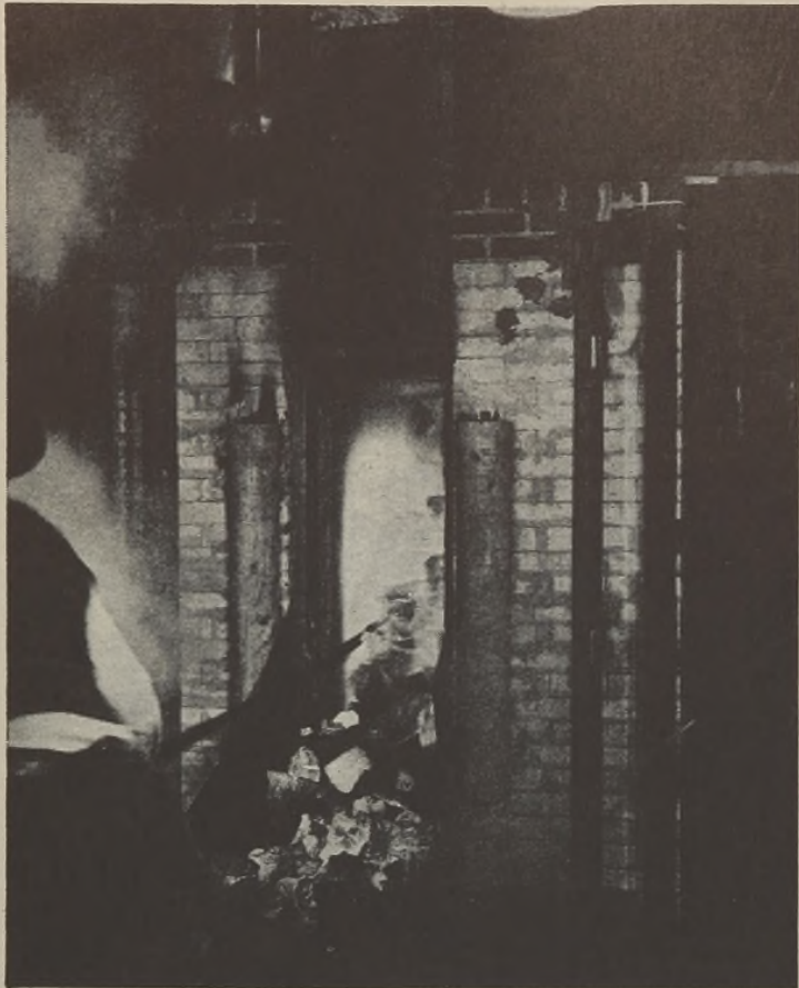
Figure 1. Discharging and Quenching Coke from Slot-Type Experimental Oven
