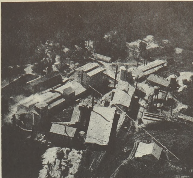
An Aerial View of a Plant of the Floridin Company, Quincy, Fla. Here Bauxite, Which Early in the War Was an Important Dehydrogenation Catalyst, Is Milled and Processed
