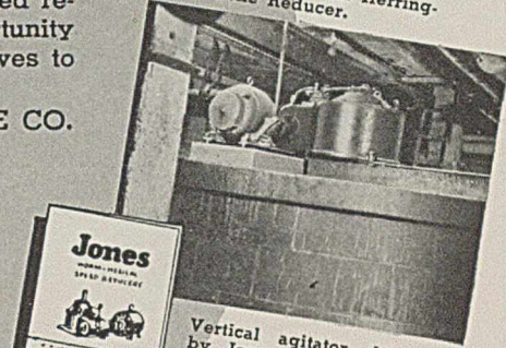
Vertical agitator driven through Jones double reduction Herringbone Reducer.
