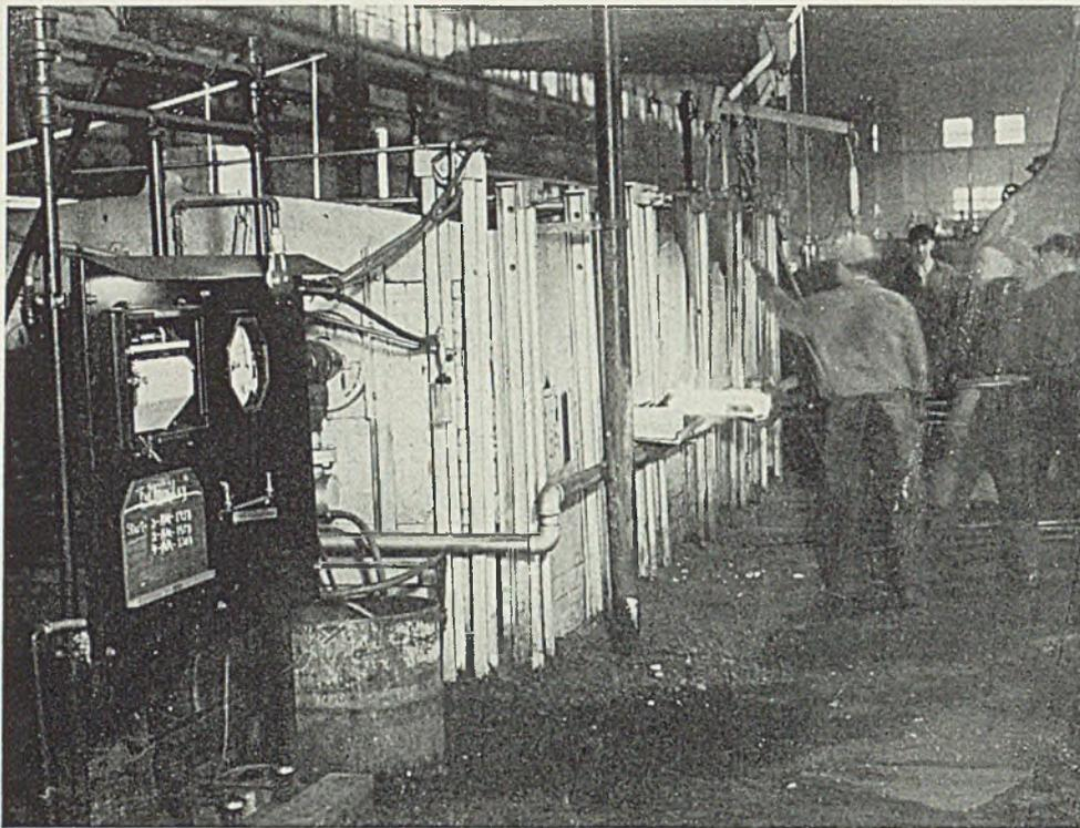
*Control instruments are set on a specially mounted board close to the furnace and in full sight of the hammer crew*
