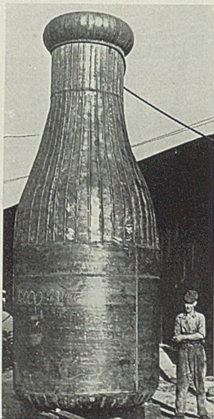
THIS STEEL BOTTLE, manufactured by Webb City and Carterville Foundry & Machine Works, Webb City, Mo., is 17½ feet high, 6 feet 5 inches in diameter in the lower portion and weighs 1600 pounds. It is located on a tower at a dairy near Jefferson City, Mo., and is painted white to the cream line, with the lower portion bearing the name of the dairy. It was fabricated from No. 12 gage steel sheets and formed by using a circular steel band which was placed at the base and raised as the welders progressed with the closing of the joints. Formation of the neck was effected by solving a simple geometrical problem, translating this solution into a chalk lay-out on the office floor and cutting the necks for the strip in accordance with the lay-out
