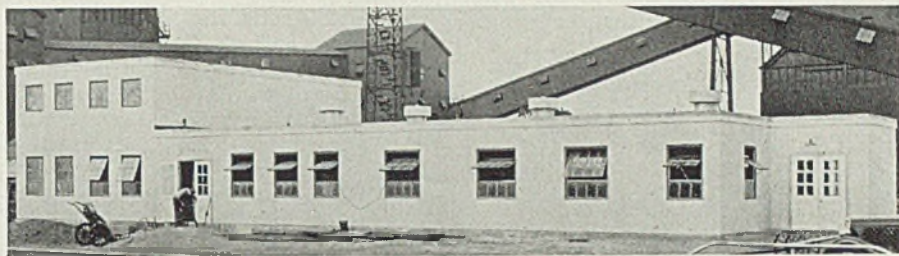
Prefabricated frameless steel office and storage building, 40 by 90 feet, erected at Hamilton, O.
