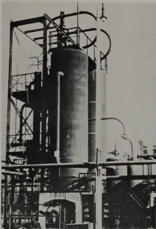
FIG. 4. CONTINUOUS BLOWING PLANT.
