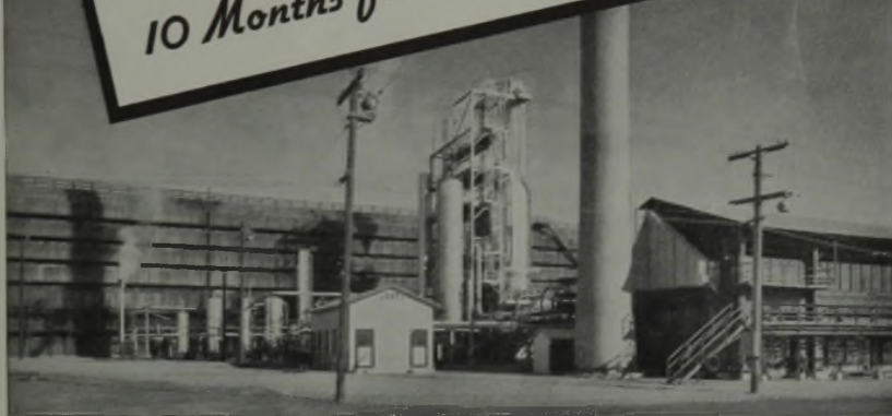
14,000 barrel per day cracking unit with visbreaking and gas oil cracking. Designed and built by Lummus
