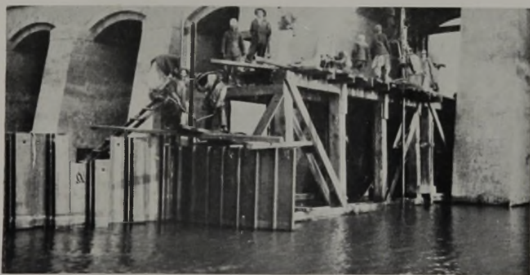
FIG. 5. ASSIUT DAM, SHOWING EMULSION BEING INJECTED.
