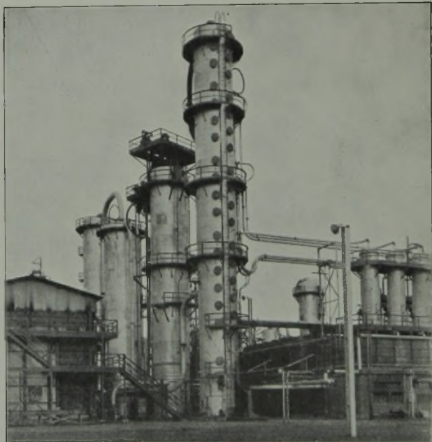
Combined Distillation and High- and Low-Temperature Cracking Unit with Vacuum Flash Tower for Residue, running 8900 barrels of crude per day.
