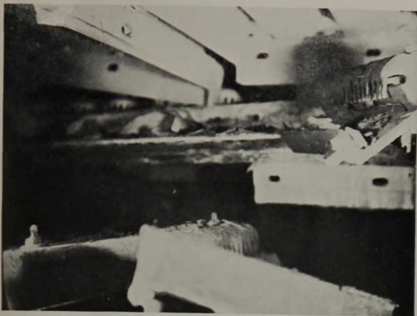
FIG. 1. RESULT OF EXPLOSION IN FRACTIONATING COLUMN.
