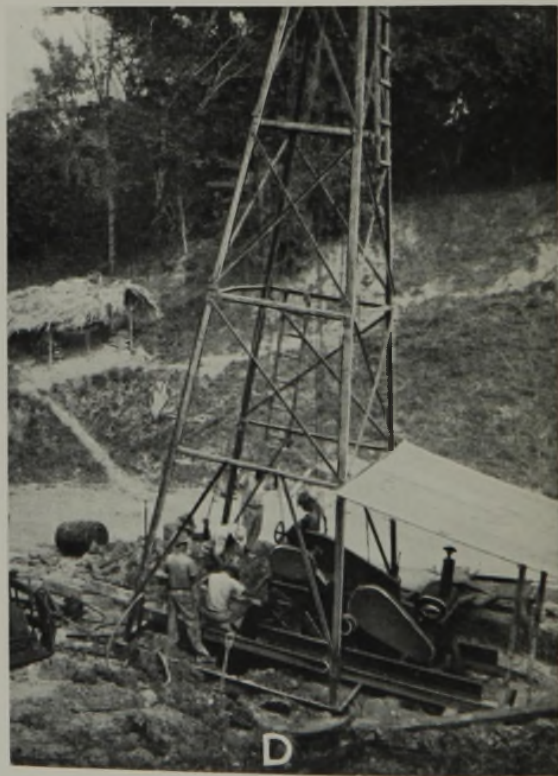
1000 FT. CAPACITY DRILLING RIG, SHOWING LOCALLY FABRICATED DERRICK DRILLING IN MONE DIABLO QUARRY TRINIDAD.
