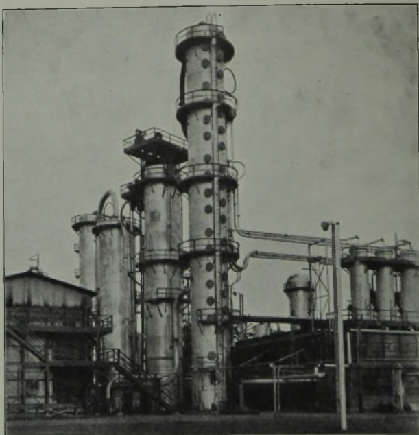
Combined Distillation and High- and Low-Temperature Cracking Unit with Vacuum Flash Tower for Residue, running 8900 barrels of crude per day.
