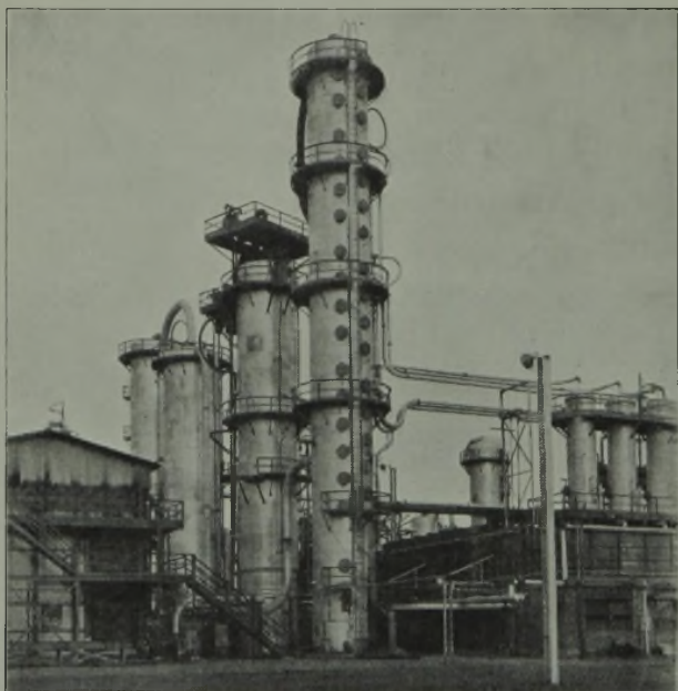
Combined Distillation and High- and Low-Temperature Cracking Unit with Vacuum Flash Tower for Residue, running 8900 barrels of crude per day.
