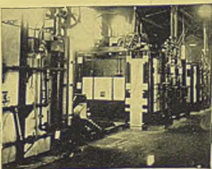
Completely automatic installation—heat treating axles.
