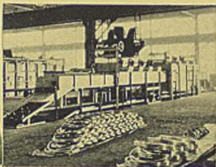
Bright annealing copper tubing in coils and straight lengths.
