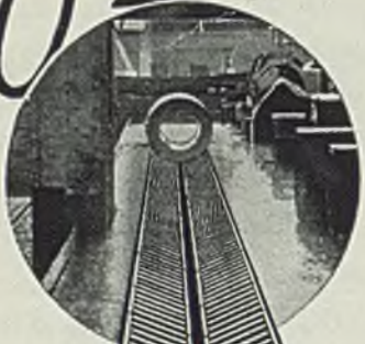
View of Trough Rolls coming from pickler with scale section and tilting sections inserted in the line of conveyor.
