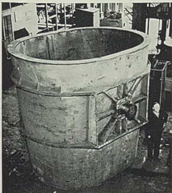
Welded steel ladle designed to handle open-hearth melts which were increased from 100 to 125 tons. Capacity of the ladle was increased by making horizontal cross sections elliptical rather than circular
