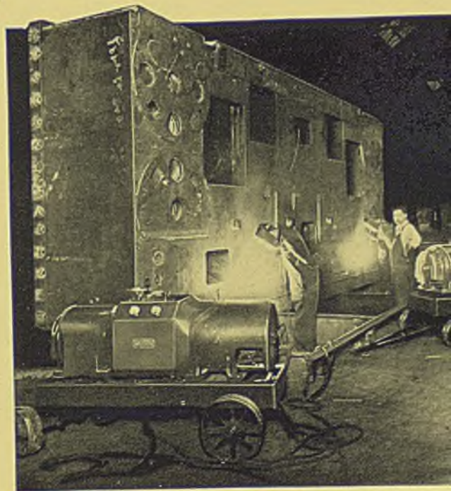
Welding on the actuator base in progress showing the battery of WILSON ARC WELDERS which serve the shop.
