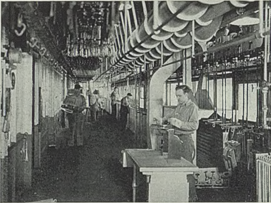
Nickel plating is done in automatic plating equipment and a maximum use is made of conveyor equipment. The inspector at the right is examining a cabinet as it comes from the plating bath
