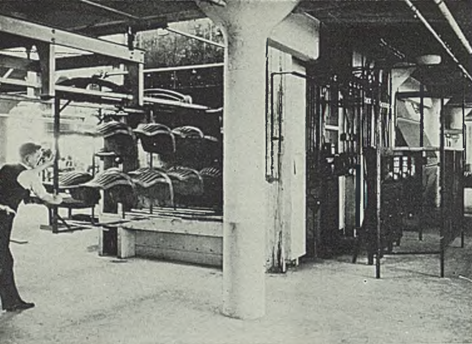
FIG. 4—Heat treating is done in special furnaces equipped with elaborate means for controlling the temperature. After being brought up to the correct heat the parts are air quenched
