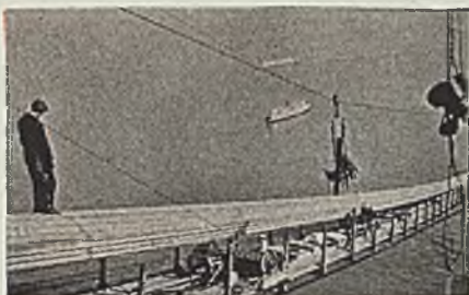
1935 Cables for the west suspension span, spun into 37 individual strands, completed and ready for compacting.
