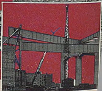
"Two of our 35-ton Speedcranes with 85 ft. booms of MAN-TEN steel successfully handled loads on the Triborough Bridge up to 37 1/2 tons at 18 ft. radius. It is estimated that the stresses resulting were in excess of 60% greater than those for which the boom was designed. This is indeed a tribute to the quality of MAN-TEN Steel." (Forsythe Equipment Co., New York.)
