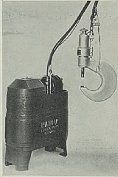
Hanna electric-hydraulic riveter furnished in portable and stationary models
