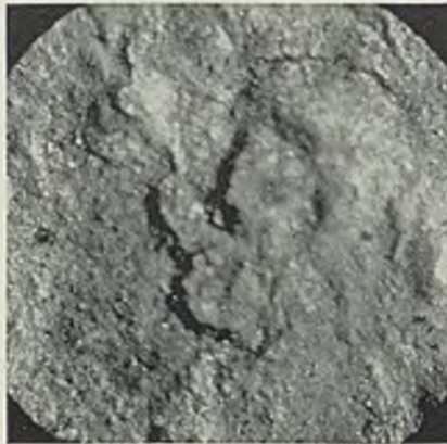
Steel painted with standard red lead, two coats, and standard aluminum paint, one coat, after 744 hours exposure to salt spray. X100
