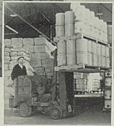
Baker Fork Trucks are built in capacities from 2000 to 8500 lbs., in tilting, non-tilting, telescoping and tilting-telescoping models.
