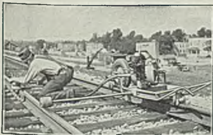
Outrigger rail grinder equipped with 5-horsepower gas engine built by the Mall Tool Co.
