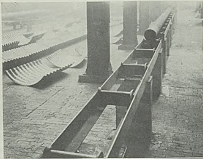
FIG. 1 (above)—A 1100-foot gravity conveyor which handles steel pipe sections 40 feet long and weighing up to 9600 pounds each. Fig. 2 (right)—Use of this conveyor table is said to have effected savings in the shearing of strip. Photos courtesy Mathews Conveyor Co.
