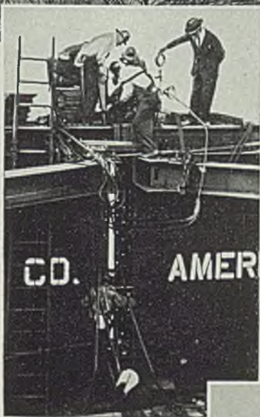
Opening at the crown, controlled by jacks, ready for the insertion of the 2 ft. 6 in. "keystone" piece which closed the arch.
