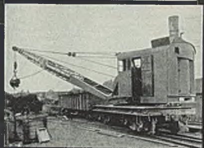
25 TON STEAM CRANE
