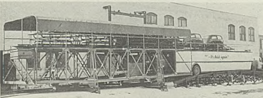
FIG. 5 (right)—Transfer car delivering bodies from two decks—by gravity from the upper deck and manually through a side door from the lower deck. Inside the plant, bodies are stored by a small tractor
