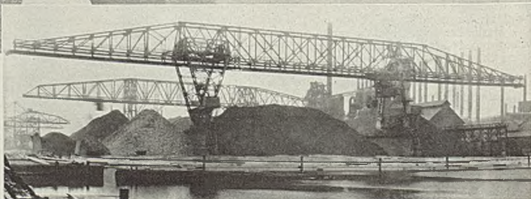
Each of the three Industrial Brownhoist car dumpers shown above will dump 120 tons of coal per minute. The bridge crane, at the right, has a bucket capacity of 15 tons of ore.
