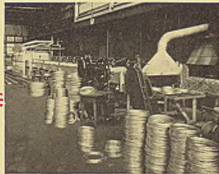
Gas Fired Radiant Tube Furnace equipped for special atmosphere for bright annealing copper tubing.
