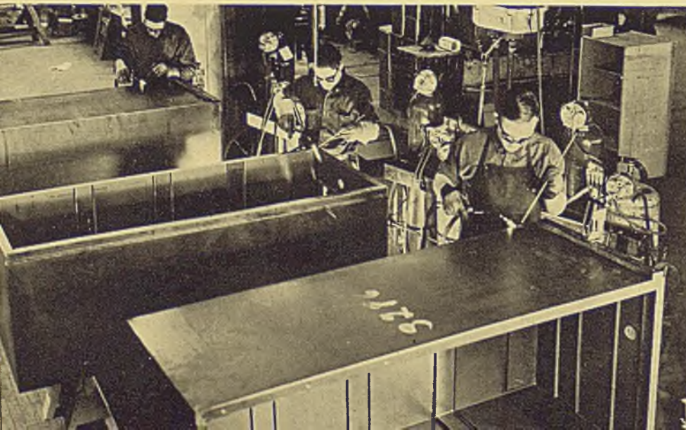
■ In assembling soda fountains at its Grand Haven, Mich., plant, Bastian - Blessing Co., Chicago, employs electric arc and oxyacetylene welding, despite the fact that the company manufactures a line of gas cutting and welding equipment. The gas welding unit used on production work on soda fountains and freezer equipment consists of a light-weight torch with 2-stage regulator and a gas economizer
