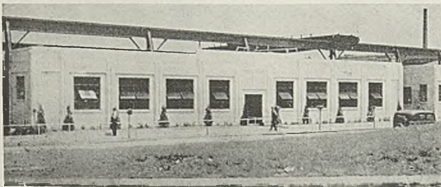
Power plant of the Schiavone-Bonomo scrap preparation yards in Newark, N. J. Photo courtesy Esso Oilways
