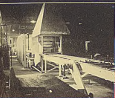
Bright Annealing Steel Tubing—continuous—5 to 25 foot lengths—2,000 pounds per hour.
