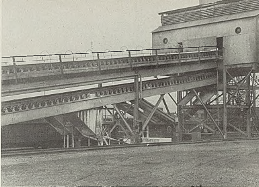
T HIS partial broadside view of the upper half of the machine and the head house shows the solid concrete deck which separates the forward and return strands
