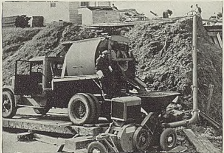
Rex Pumpcrete, first machine to pump concrete in America, made by Chain Belt Company, Milwaukee. Vital parts of the Pumpcrete, notably Valve Plugs and Valve Chambers, are Vanadium Cast Steel, furnished by Sivyer Steel Castings Company, Milwaukee.
