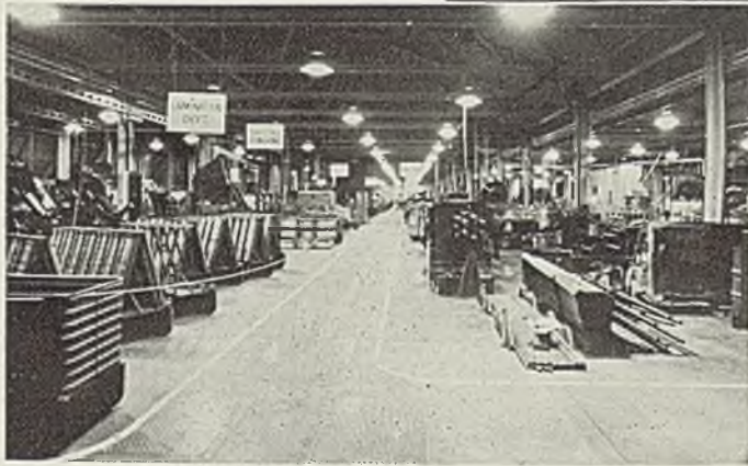
This view of the plant was taken at night. Note well marked aisles and neatly arranged skid loads of laminations
