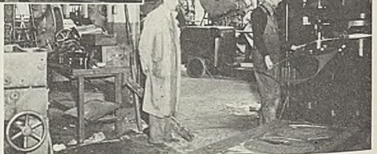
14 —An adequate sheet metal department is in operation as all the bodies are made on the job. At right is a partial view of this department with one of the larger presses in at the right foreground. This press is a product of the Cleveland Punch & Shear Co.
