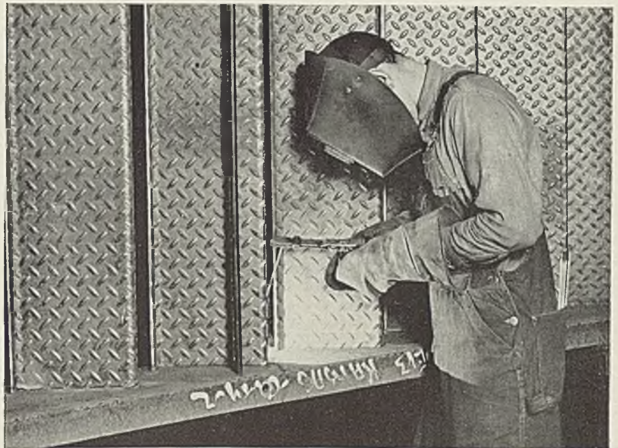
Courtesy Builders Steel Co., North Kansas City, Mo.
