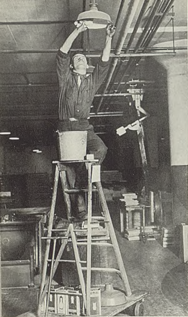
Monthly cleaning of light reflectors by a trained maintenance man is a profitable procedure both from the standpoint of lighting cost and working efficiency
