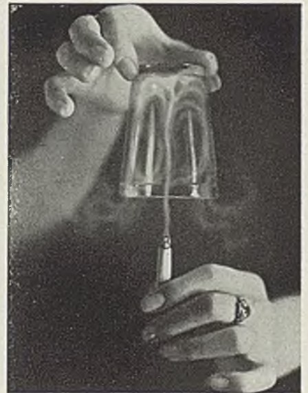
Fig. 3—Principle of natural circulation demonstrated by smoke and inverted tumbler
