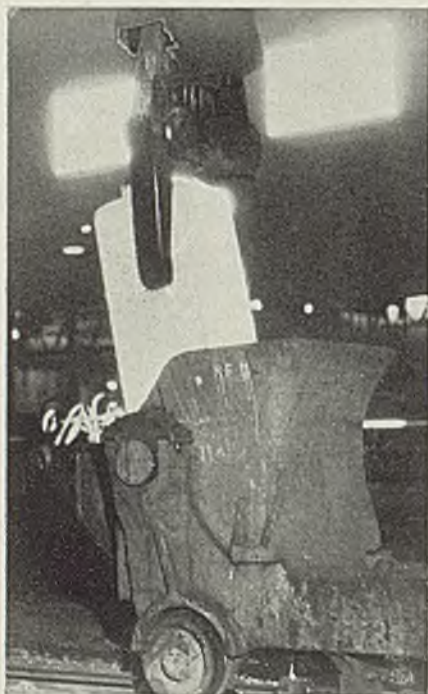
Fig. 1—Freshly drawn ingot being placed on chariot for delivery to blooming mill
