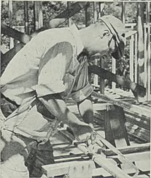
Floor joists are placed on the sills which are lined on the foundation walls. Floor slabs, of heavy nailing concrete, are nailed to joists
