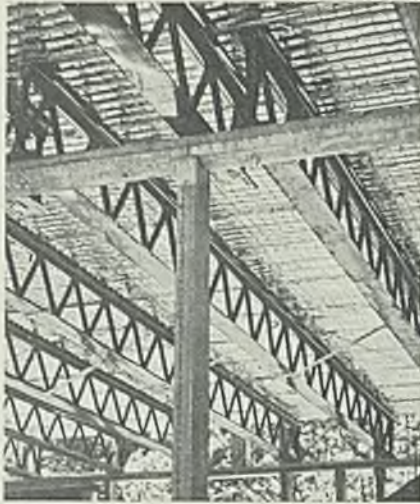
View upward from first floor, showing construction details of joists and flooring above
