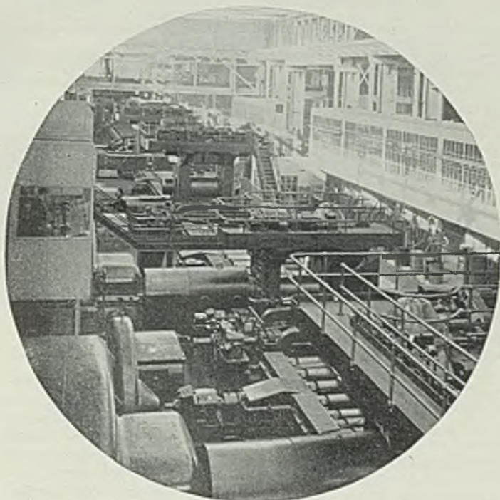
Roughing mill which comprises one stand of 2-high and two stands of 4-high rolls. Each of these stands is preceded by edging rolls
